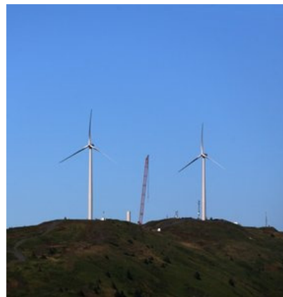
Each of these turbines produces up to 1.5 MW of electricity
