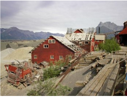
Kennecott Leach and Flotation Facility
